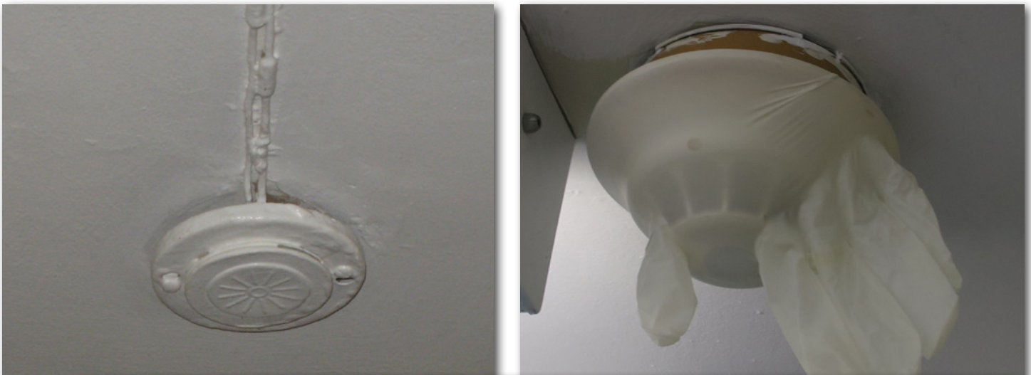
Figure 34. Fire safety systems should be frequently inspected and tested during this period, ensuring they are not damaged by construction activities (e.g., heat detectors painted, or smoke detectors covered, to limit false alarms due to dust and debris).
