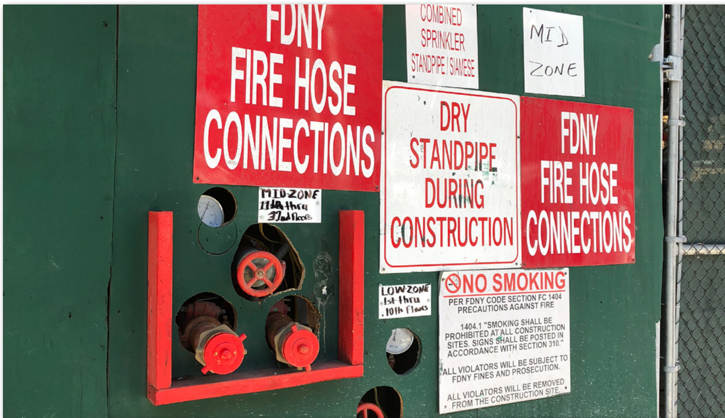
Figure 36. Temporary measures during restoration and construction should be clearly marked and simple to understand. ©Marrion Fire & Risk Consulting PE LLC-Chris Marrion
